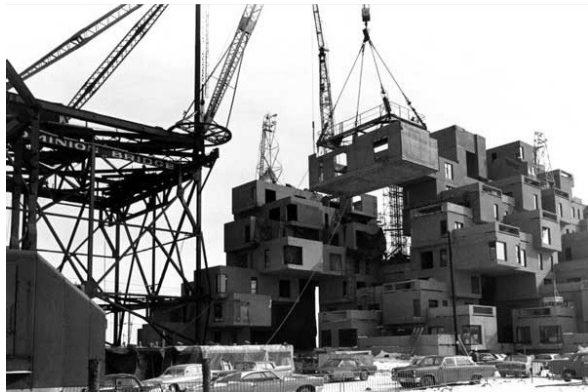
Figure 9. Assembling of Habitat'67, Montreal, 1967. Available at: < https://www.archdaily.com/404803/ad-classics-habitat-67-moshe-safdie/51e85669e8e44e33c300001d-ad-classics-habitat-67-moshe-safdie-image >. Accessed: 19 Nov 2017.
