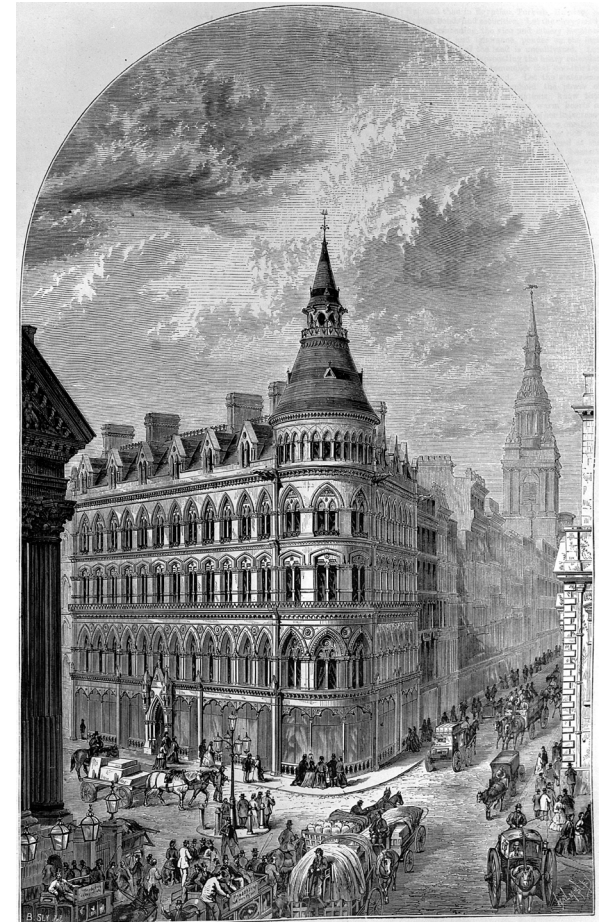
Figure 8. Mappin and Webb building, illustrated in the Builder , 1871. Source: RIBA Collections.
