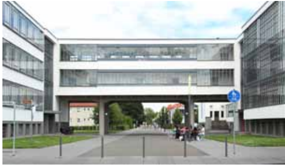
Figura 4 Visão do edifício Bauhaus Dessau a partir da Gropius-sallee. Fonte: Megan Sveiven. “AD Classics: Dessau Bauhaus / Walter Gropius” 10 Nov 2010. ArchDaily. Accessed 2 Dec 2015. http://www.archdaily.com/87728/ad-classics-dessau-bauhaus-walter-gropius/
