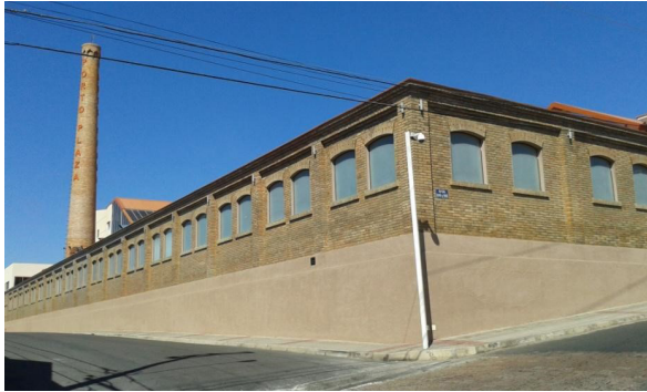
Figure 10. Lateral view of the textile factory. Source: Deborah Neves, 2013.
