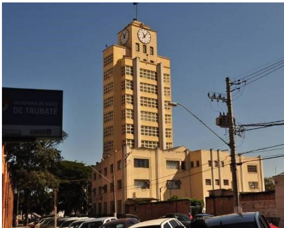
Figure 6. Offices' building. Source: Deborah Neves, 2012
