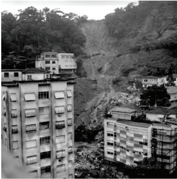
Figure 8. Photo of the landslide in 1967. Source: O GLOBO (2013).
