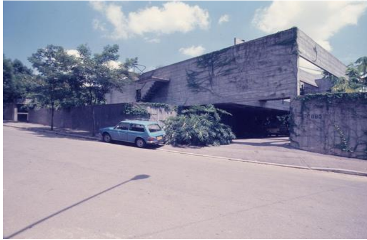
Figure 9. Fernando Millan's Residence, Morumbi, São Paulo. Project by Paulo Mendes da Rocha, 1970. Photograph: Hugo Segawa. FAUUSP Library Archives.
