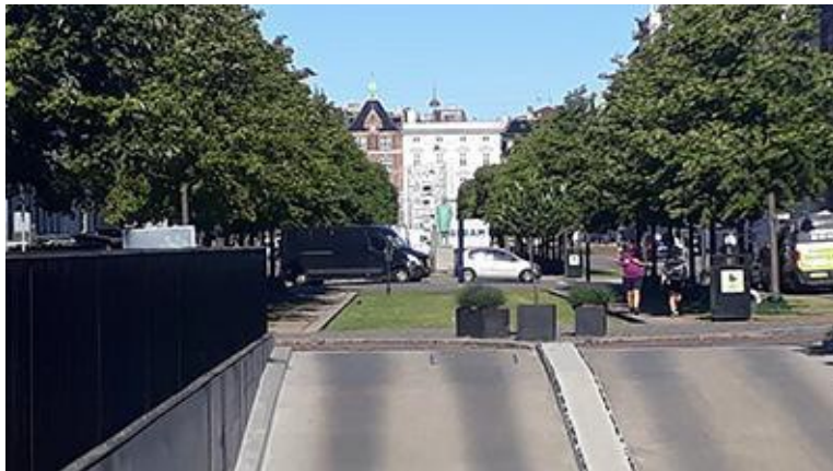
Figure 1. St Annæ Plads, the lowered central boulevard doubles up as a rain collector in flash flooding.
