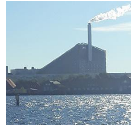
Figure 3 Copenhill (Amager Bakke) by BIG Architects. A Waste-to-Energy Plant with roof top artificial ski slope.
