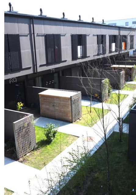
Figure 6. “Grøndalsvænge” is designed by OVN Architects and is located in Copenhagen (Denmark). Source: Personal Collection.
