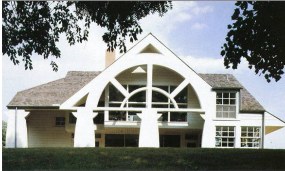
Figura 12. Fachada da Casa em Delaware. Fonte: The Architectural Archives, University of Pennsylvania by the gift of Robert Venturi and Denise Scott Brown. Foto: Matt Wargo.
