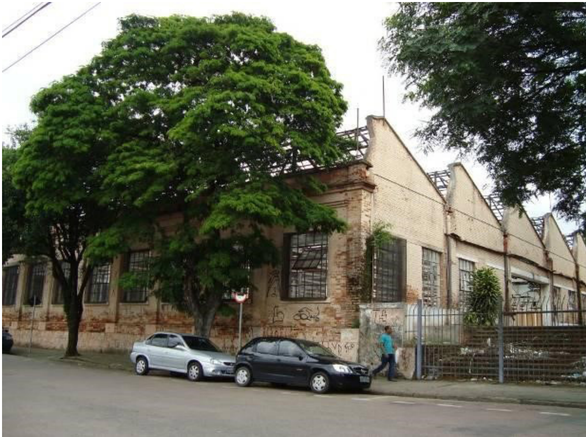
Figure 9. Frontal and lateral façade views. Source: José A.C.Zagato, 2011.
