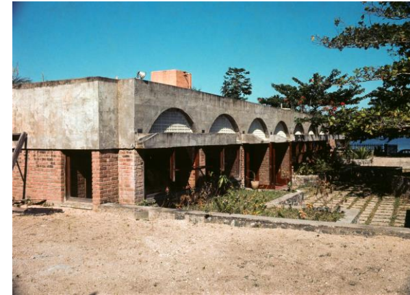
Figure 8. Simon Fausto's Residence, Ubatuba. Project by Flávio Império, 1961. Photograph: Benedito Lima de Toledo. Flávio Império Archives - IEB USP. Available at http://www.flavioimperio.com.br/galeria/505589/509929
